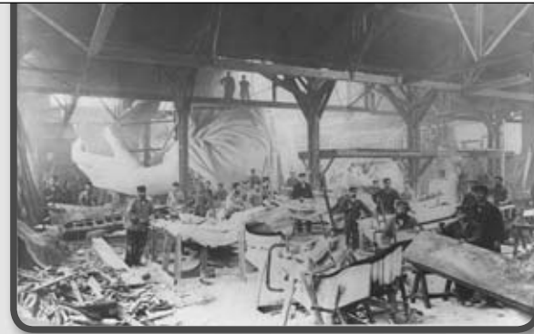
➡ Bartholdi used scaffolding to hold the parts of the statue in place while he worked.
